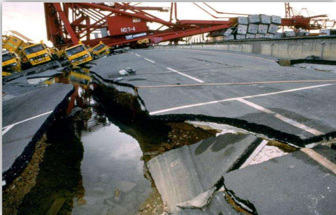
FIGURE 22 : DAMAGED KOBE ROUTE OF THE HANSHIN EXPRESS WAY
